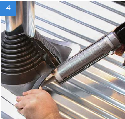
4 Apply the sealant to the area between the flange and the roof surface.
