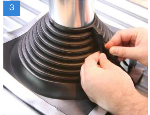
3 Secure Master Flash® Retrofit around the pipe using the plastic clamps provided to seal the flange.
