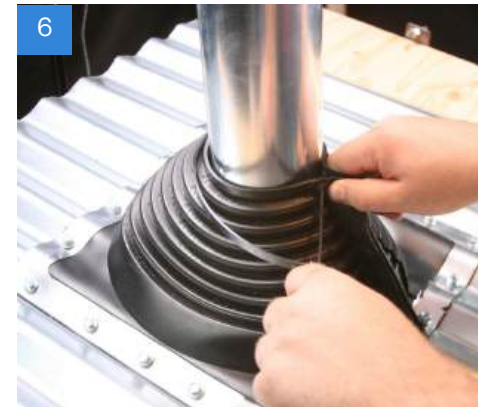
6 Drill holes in the flange for the fastening strap. Thread the strap through the hole. Tighten the fastening strap securely to ensure a proper seal. Additional sealant can be applied between the flange and the pipe.
