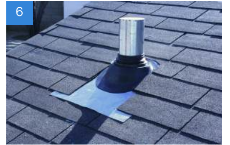
6 Finish installing the roof around the roof flashing.
