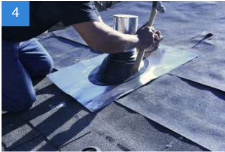
4 Secure the metal base with nails and a hammer.
