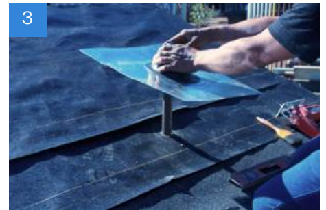
3 Slide the flange onto the pipe.
