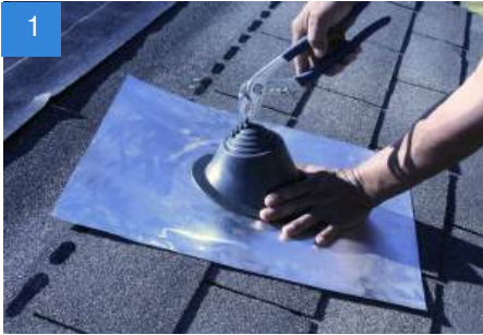
1 Adjust the flashing to the correct pipe diameter.
