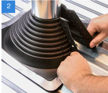
2 Slide Master Flash® Retrofit sideways onto the pipe.
