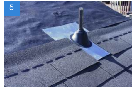
5 Install the roof tiles along the sides of the Master Flash®.
