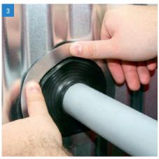
Press Master Flash® Low Profile down, bending it to conform to roof profile or irregularities. A blunt tool will help to form flashing to tight roof angles.
