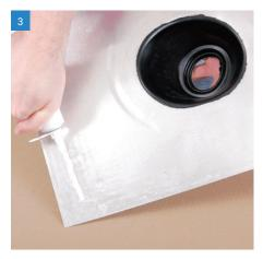
Apply sealant on the underneath of the metal base
