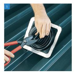
Select an appropriate Master Flash® Standard with a pipe range that goes below and beyond fitting. If necessary, use the lines clearly shown on the flashing to trim an opening 20 - 30% smaller than pipe diameter. For the steep roof slopes or higher corrugation of the profile, bigger size of Master Flash® should be chosen.
