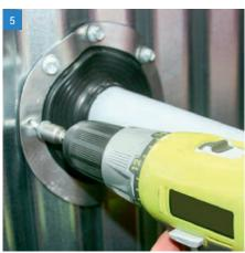
Use fasteners to complete sealing. For a secure installation, fastener spacing must not exceed 1.5" (38 mm)
