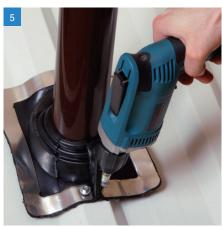
Use fasteners to complete sealing. For installation, fastener spacing must not exceed 1.5" (38 mm).
