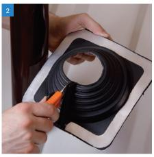
If using this product as a Retrofit, cut down the side in the clearly-marked flange.
