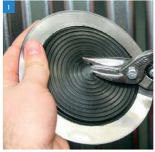
Select an appropriate Master Flash® Low Profile with a pipe range that goes below and beyond fitting. If necessary, use the lines clearly shown on the flashing to trim an opening 20-30% smaller than pipe diameter.
