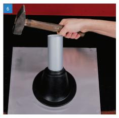
Secure and fasten the metal base to the roof.
