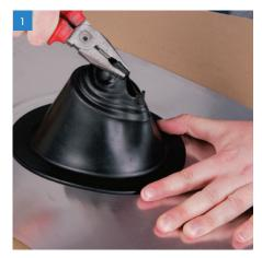
Select an appropriate Master Flash® Residential with a pipe range that goes below and beyond fitting. If necessary, follow the lines clearly shown on the flashing and use pliers to pull the tab to create an opening 20 - 30% smaller than pipe diameter. For the steep roof slopes or higher corrugation of the profile, bigger size of Master Flash® should be chosen.
