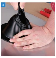
Finish adjustments to flashing opening by hand.
