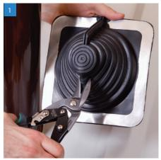
Select an appropriate Master Flash® Multi-Flash with a pipe range that goes below and beyond fitting. If necessary, follow the lines clearly shown on the flashing and create an opening 20-30% smaller than pipe diameter. For the steep roof slopes or higher corrugation of the profile, bigger size of Master Flash® should be chosen.
