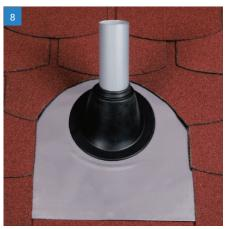
Complete installation of roof tiles over the Master Flash® Residential's metal sheet base.
