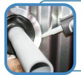
Apply sealant between the base of the flashing and the roof.
