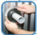
Slide the Master Flash® Low Profile down the pipe, using a non-petroleum-based lubricant to ease installation.
