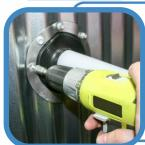
Use fasteners to complete sealing. For a secure installation, fastener spacing must not exceed 38mm (1.5").
