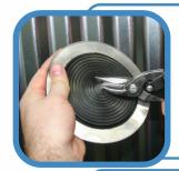
Select an appropriate Master Flash® Low Profile with a pipe range that goes below and beyond fitting. If necessary, use the lines clearly shown on the flashing to trim an opening 20-30% smaller than the pipe diameter.
