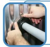
Press Master Flash® Low Profile down, bending it to conform to roof profile or irregularities. A blunt tool will help to form flashing to tight roof angles.
