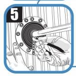
Crimp the gripper with pliers or other crimping tool to complete installation. Additional sealant may be applied onto the seam. Apply as needed.
