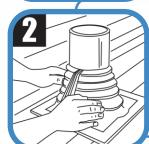
Wrap Master Flash® Retrofit around the pip and press it down, bending it to conform to roof profile or irregularities. A blunt tool will help to form flashing to tight roof angles.
